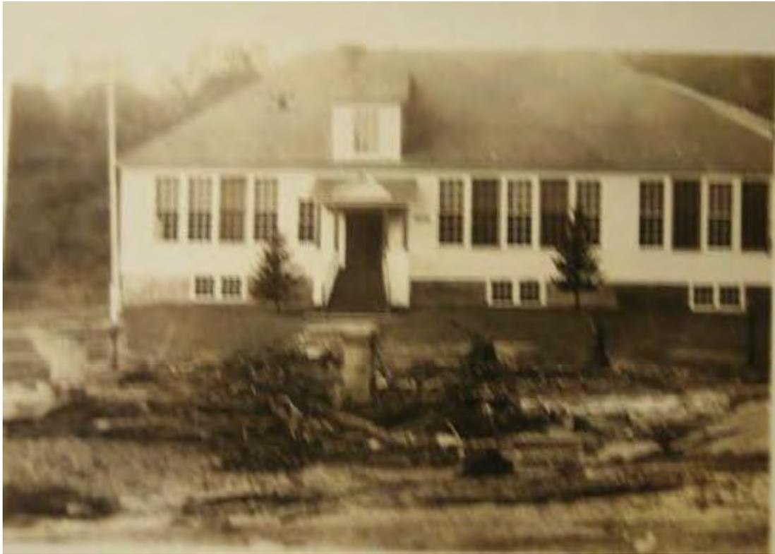
Figure 13. View southwest showing the flood damage in 1938 in front of the High School, now the Municipal Building, in Jacksonville (Bennington Museum, Bennington, Vermont. Gift of Marge Doyle, Cat No.#2004.301.7). Note that the “Welcome to Jacksonville Bridge,” built in 1926, survived the flood, but the ground around it was scoured.
